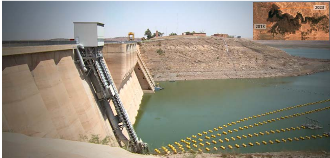
Figure 12. Photograph of Al Massira Dam in 2023 showing its lowest fill level, approximately 5.6%. Upper right: Satellite image indicating the water storage extent in 2013 and 2023.
